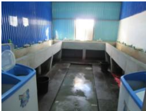
NEPC Workers Shower and Laundry Facilities
