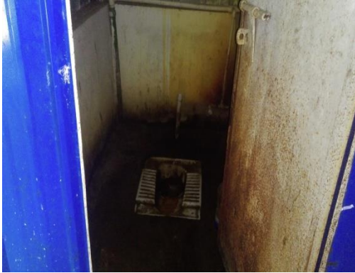
NEPC Subcontractor labors' toilets facility
