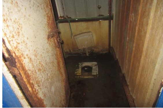
Toilet facility (NEPC)
