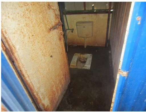
NDE Employees' Toilet Facilities
