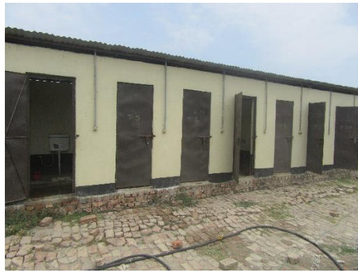
NDE Employees' Labor Shed Sanitary Conditions
